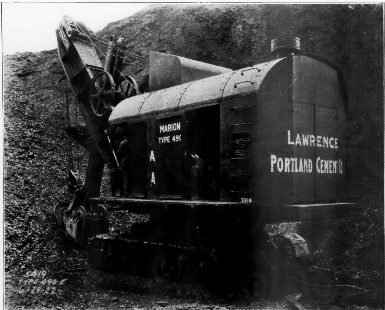
New Revolving Shovel
